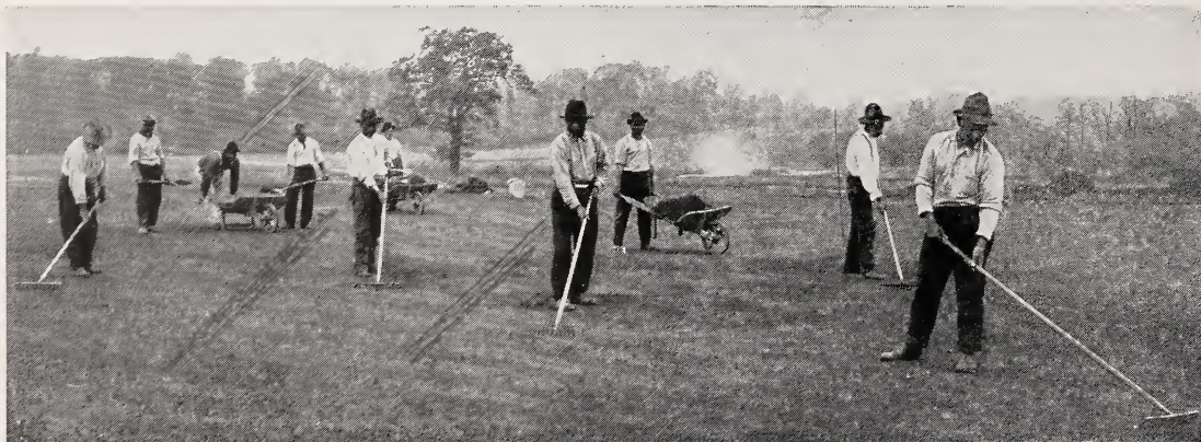
Renovating on the Nassau Country Club, L. I. Stumpp & Walter Co.'s Seeds used
